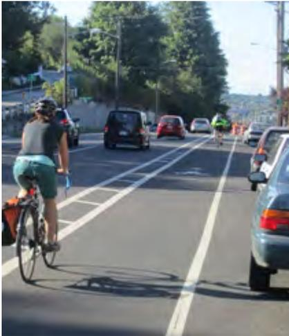
Buffered bike lane with on-street parking. The buffer separates the bike lane from the travel lane.
