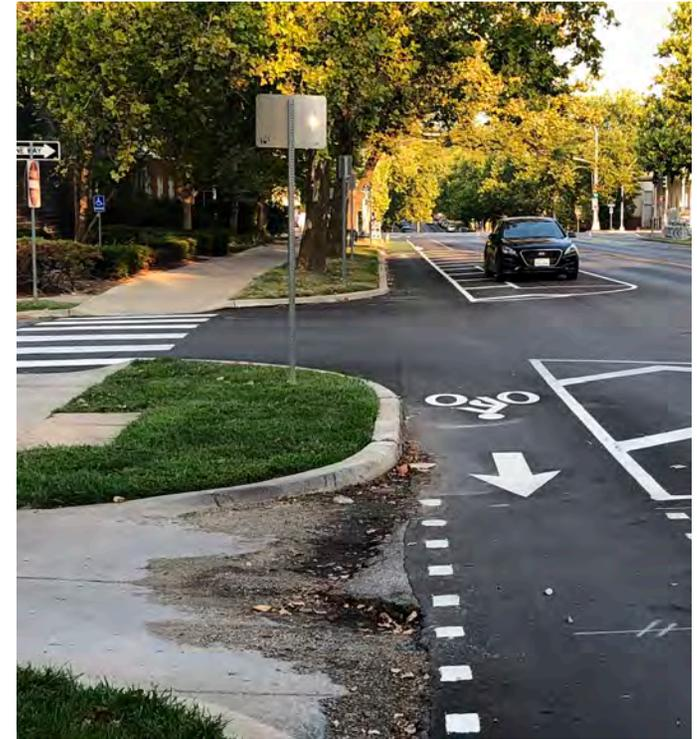
Buffered bike lane with buffer separating bicycles and on-street parking. This arrangement uses parked cars to provide additional separation. (Armour Boulevard, Kansas City, MO)
