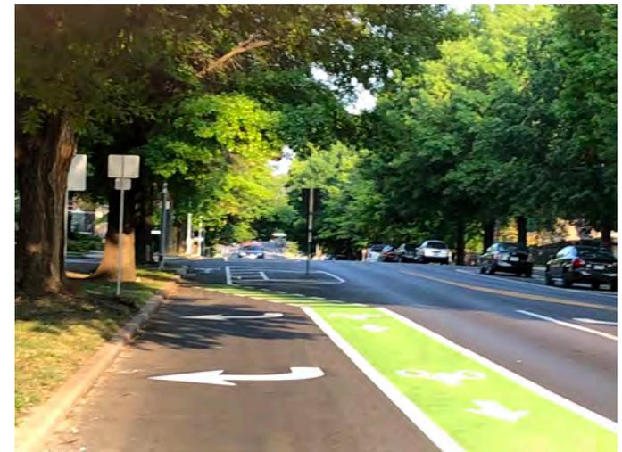
Green paint is used to mark conflict zones as motor vehicles cross the bike and buffer to make right turns.
