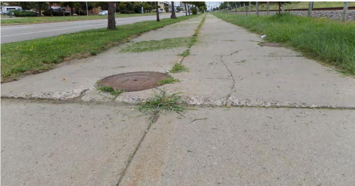
*Heaving pavement and horizontal cracking create hazards for bicyclists.*
