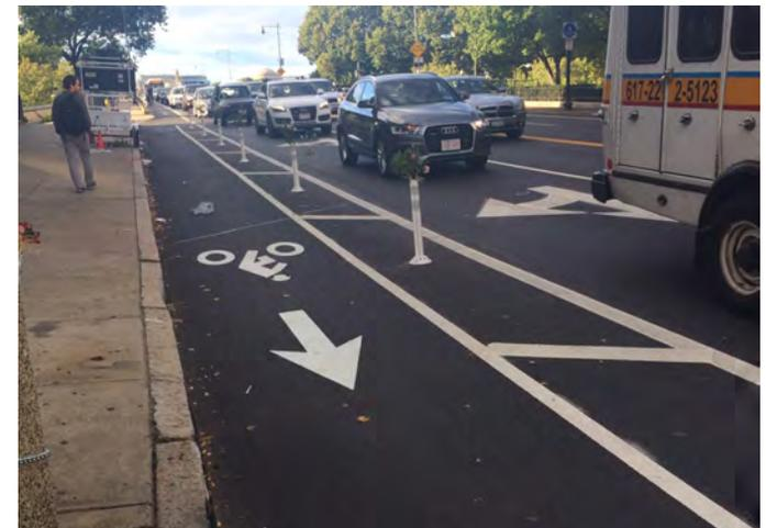
*Flexible delineators can use a variety of materials, mounting mechanisms, and spacing configurations*
