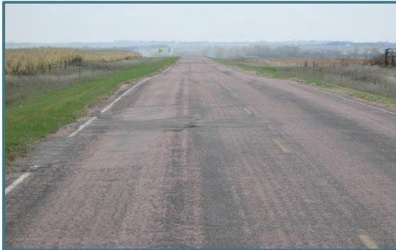
***The 1-mile segment of 448<sup>th</sup> Avenue (CH 5), between Lake County and 245<sup>th</sup> Street, is a candidate location for bituminous to gravel surface conversion. Low traffic volumes, deteriorating pavement condition, and a gravel-surfaced roadway in Lake County are all considerations.***
