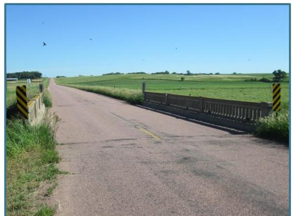
**The 448<sup>th</sup> Avenue (CH 5) bridge over the Little Vermillion River was constructed in 1940, is currently posted for load restriction, and has a sufficiency rating less than 60.**
