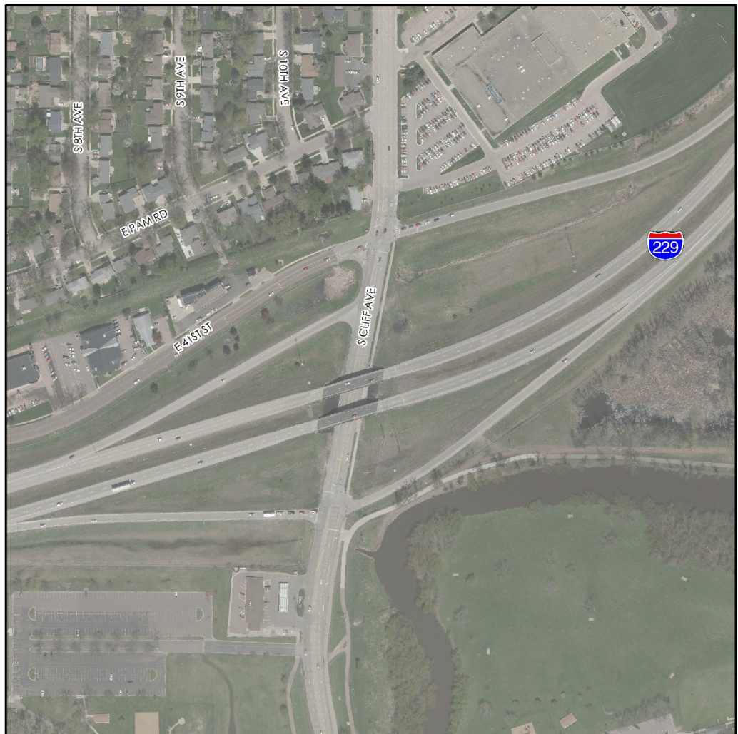
Figure 8 – Existing I-229 at Cliff Avenue Interchange
