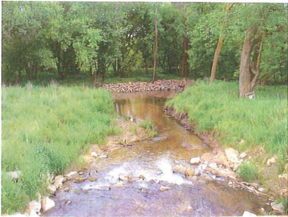
Figure 2: Downstream riprap
