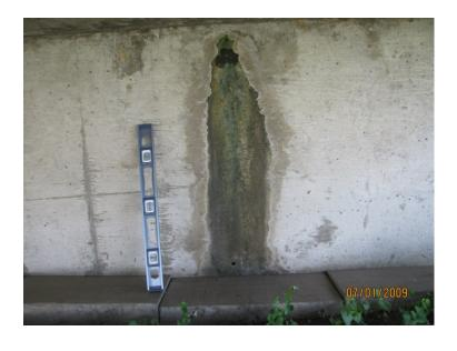
Leakage through the abutment back wall
