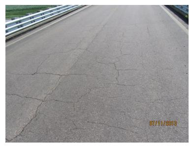
Deck overlay starting to crack and deteriorate
