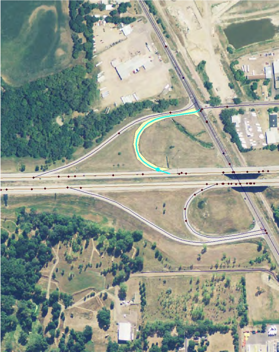
Interstate Ramp – Rice Street NB Off Ramp
