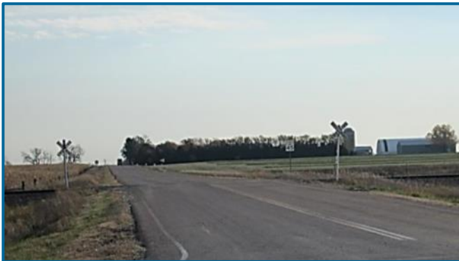
Davison County has 37 at-grade rail crossings throughout the County. Many of these crossing feature passive controls similar to the one pictured (above).
