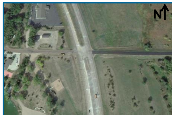
SD 37 & 251 st Street Intersection (Source: Google Earth)
