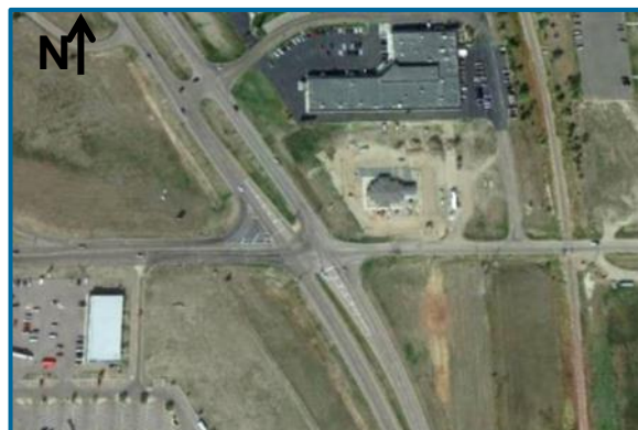
SD 37 & 255 th Street Intersection (Source: Google Earth)
