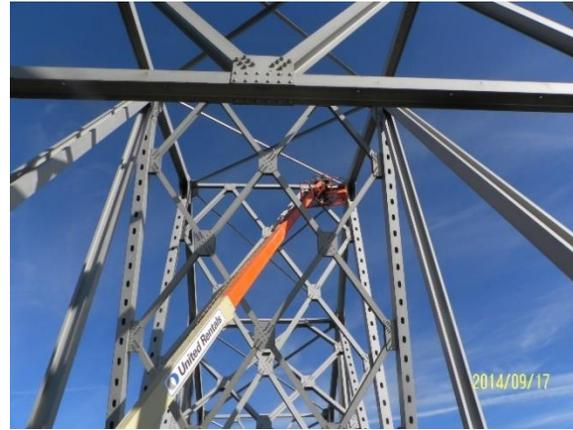
*Figure 3.22 Structure Inspections*
