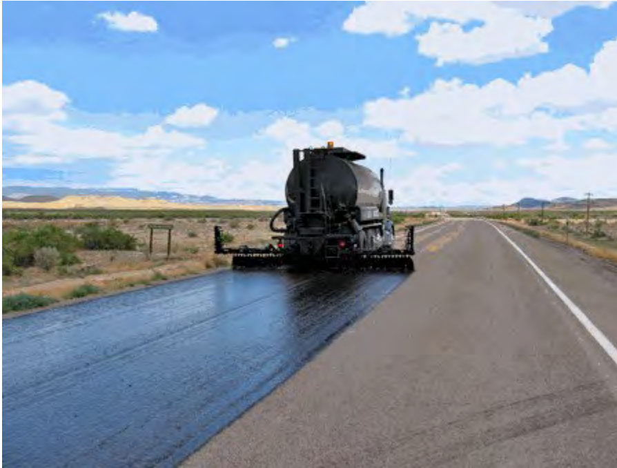
Figure 39: PASER Rating 6-7 Intervention
