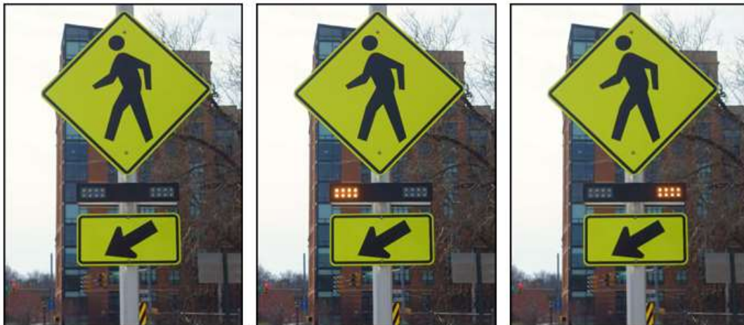
Figure 6. Example of RRFB dark (left) and illuminated during the flash period (center and right) mounted with a W11-2 sign and W16-7P plaque at an uncontrolled marked crosswalk.
