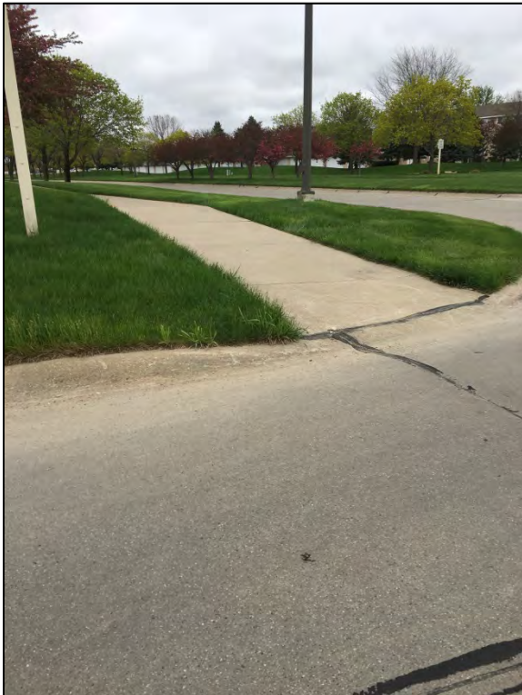
The Americans with Disabilities Act (ADA) requires specified slopes, landing areas, and tactile warning devices at intersections.
