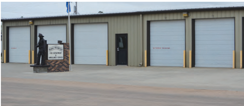
7th Street improvements in Burke will benefit its fire and ambulance services.
